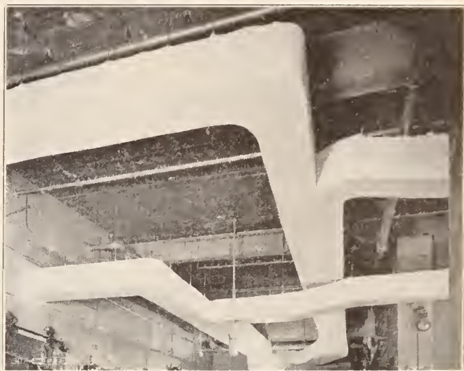
6. Plaster board ducts plastered. Note neat finish.
